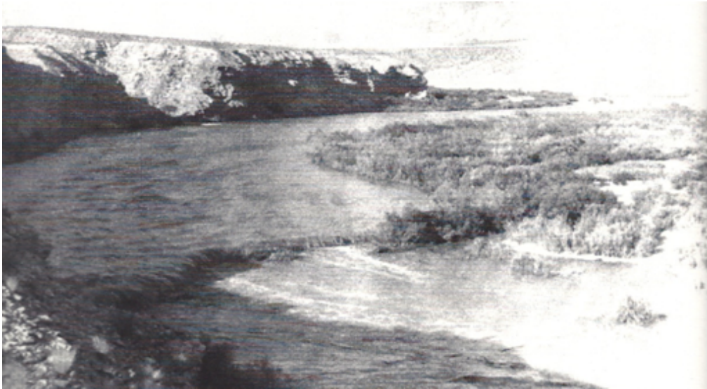
Virgin River Brush Diversion Dam, Virgin River Historical Museum
