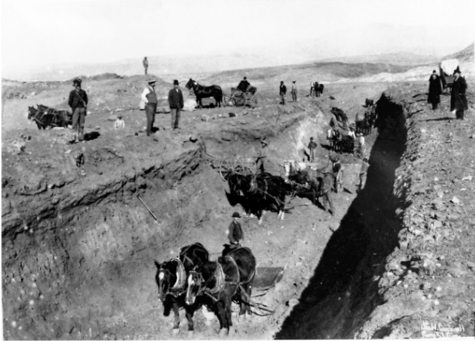
Workmen and Horse Teams Digging Washington Fields Canal, 1892, DSC Library Work on
