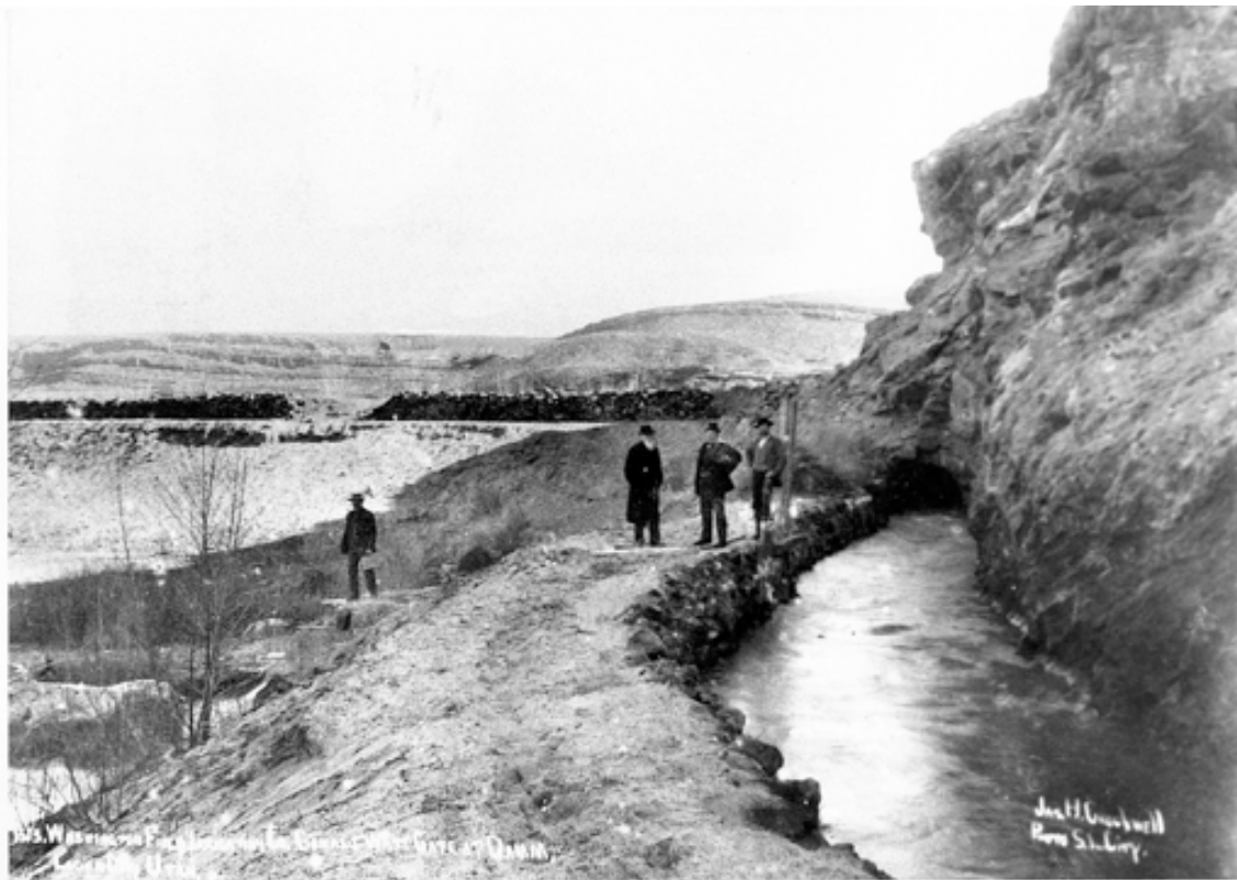
Washington and St. George Fields Canal emerging from Tunnel, 1891, DSC Library
