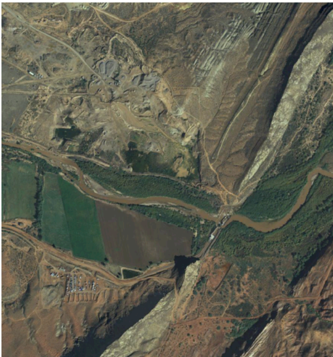
2009 Aerial Photo of Washington Fields Dam
