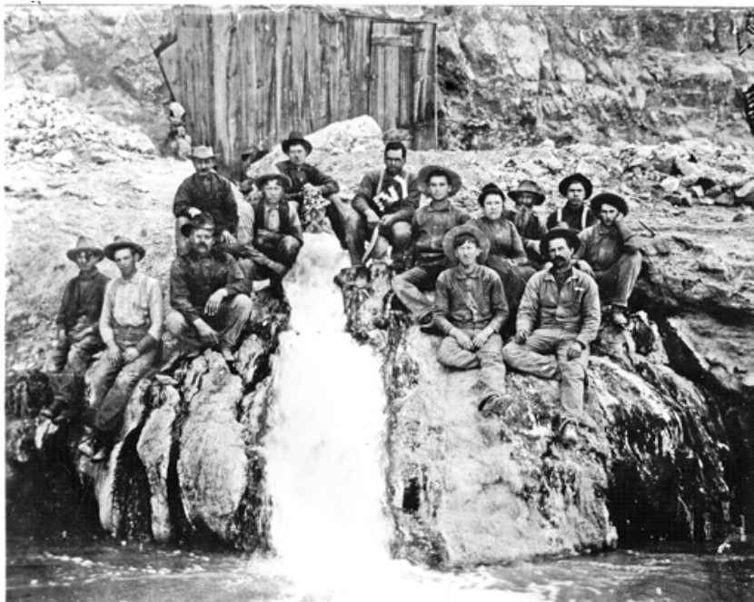
Outlet of LaVerkin Canal Tunnel with Workmen, 1890, DSC Library
