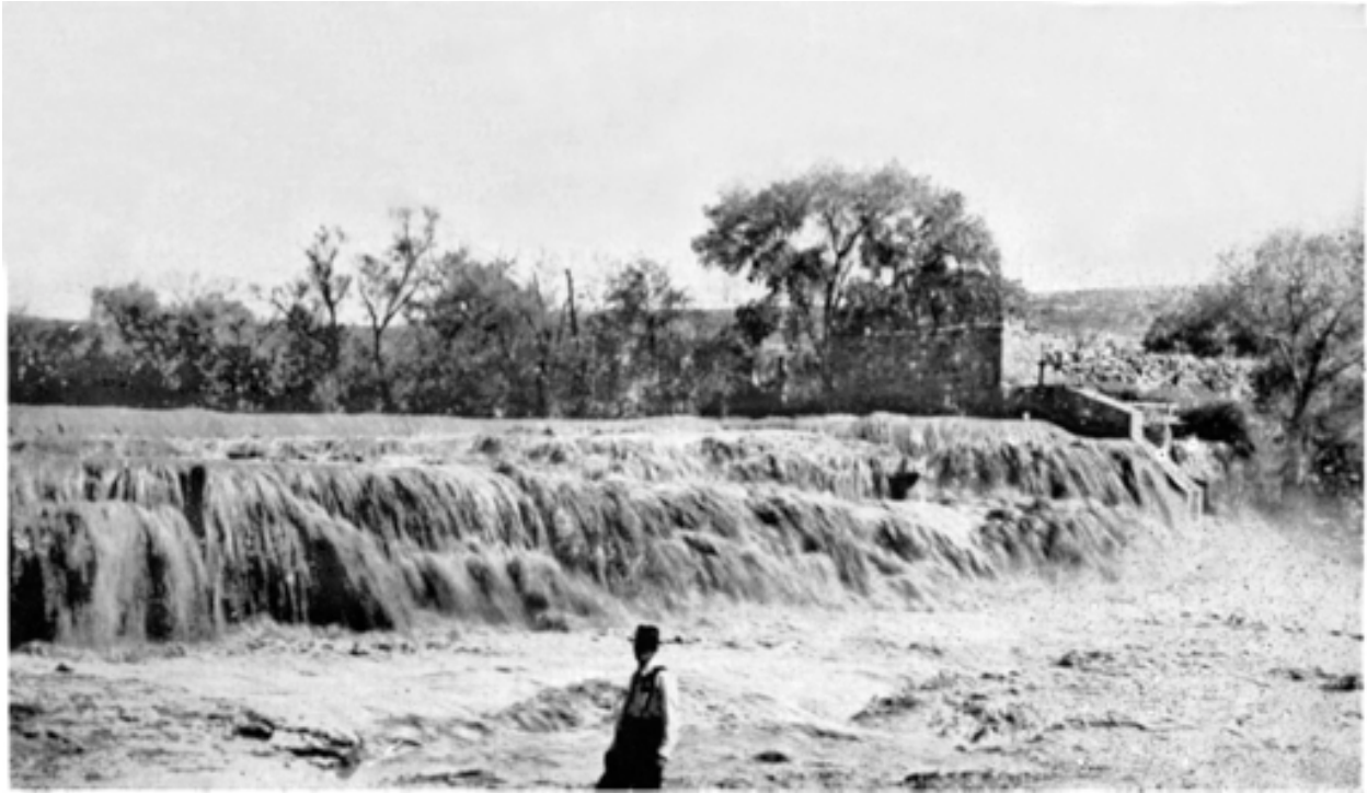
Washington Fields Dam Spillway Flood Water, DSC Library
