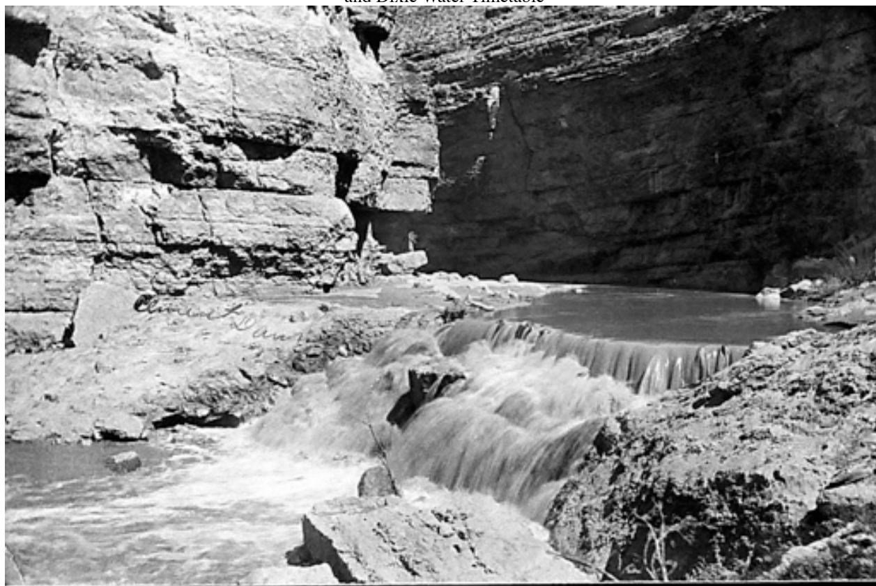
Hurricane Canal Cement Dam, DSC Library
