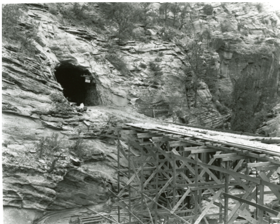
Hurricane Canal Tunnel and Bridge Construction, 1906, DSC Library
