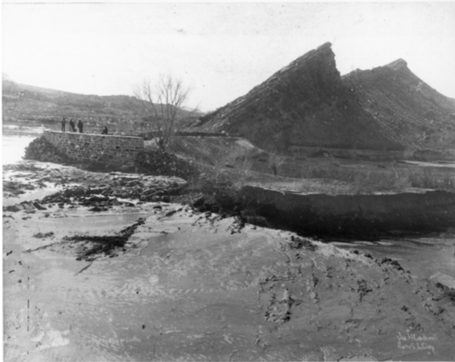
Washington Fields Dam, 1891, DSC Library
