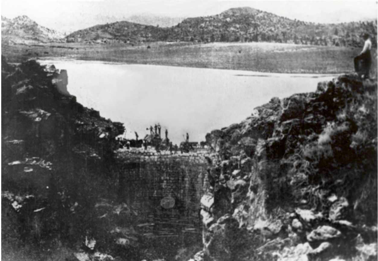
Enterprise Dam during Construction, ca. 1900, DSC Library
