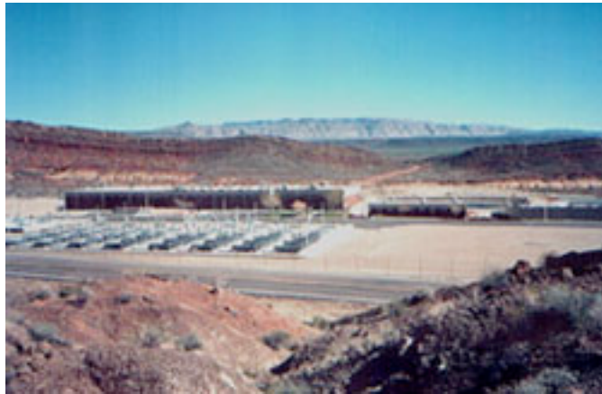
Quail Creek Water Treatment Plant, now a 20 MGD facility.
