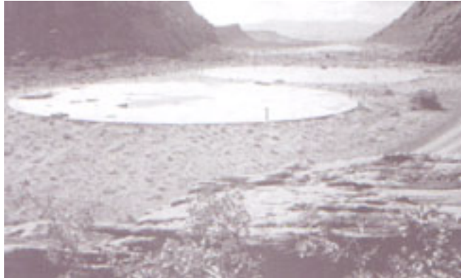
Each of these 3 million gallon, concrete tanks lies level with the landscape in Snow Canyon.
