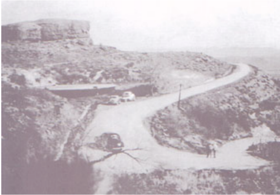
Early view of the water tank on Skyline Drive. Note the Sugar Loaf at upper left.
