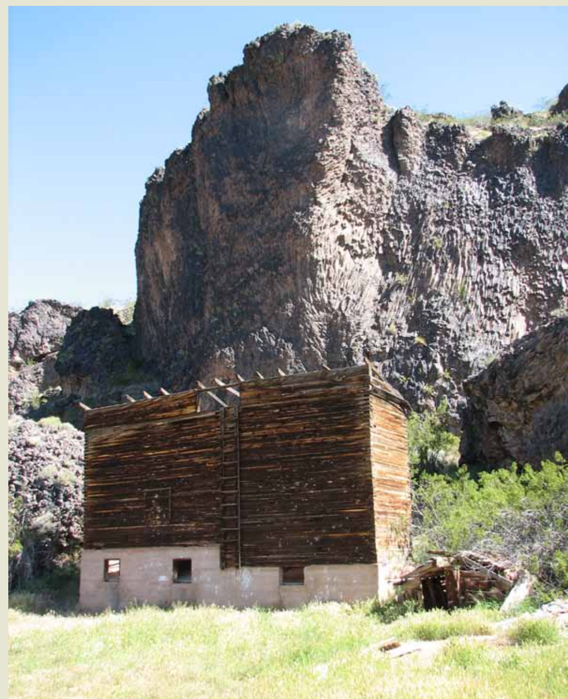
A grain storage building for the turkey farm.
