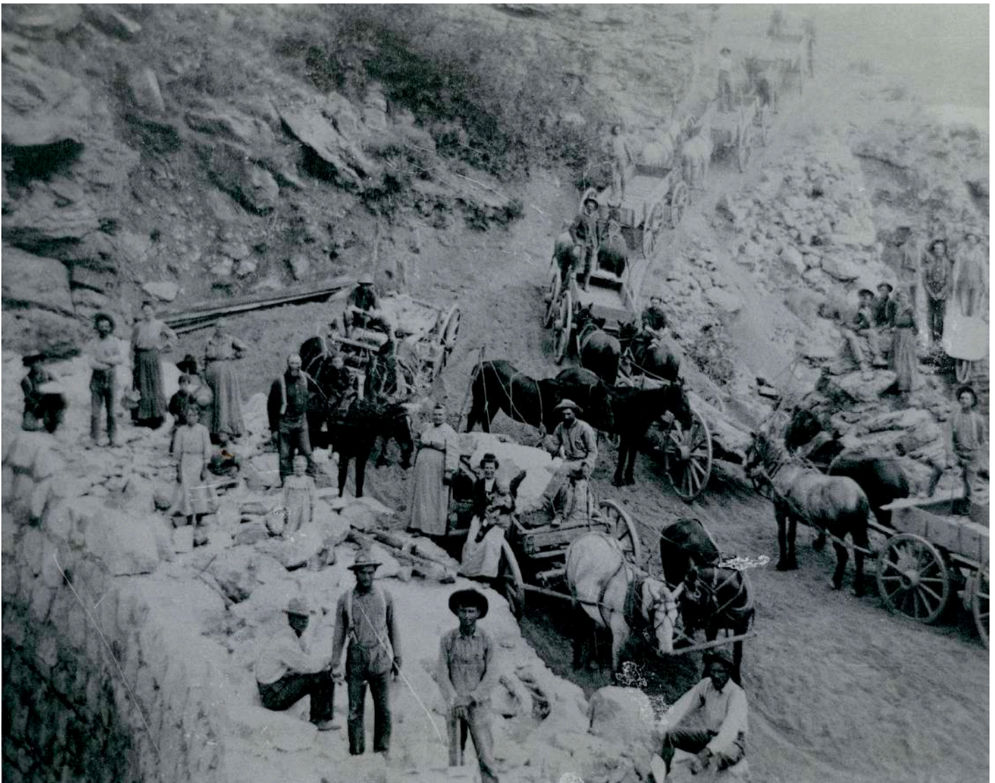
Members of the Hebron Reservoir and Irrigation Company at work on their Dam 1909
