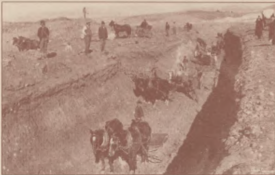
A 5 mile long canal was constructed before the water could reach the fields. It was completed by 1893.
