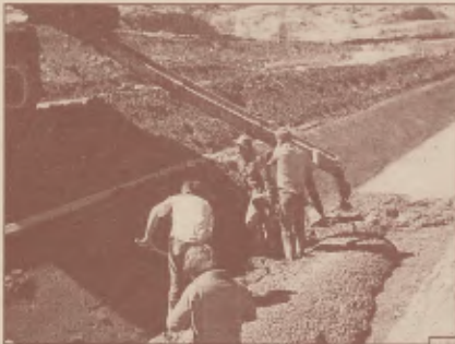
Pouring cement for the Concrete ditch.
