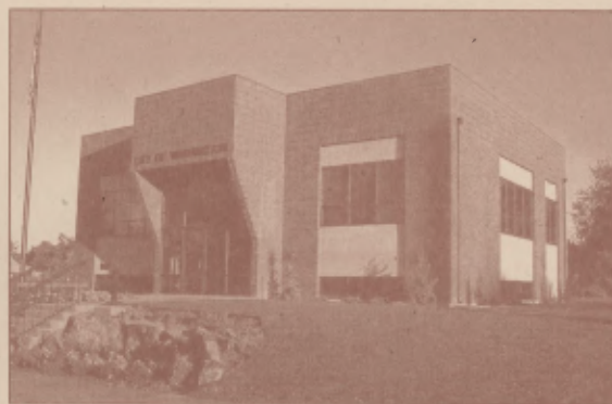
In 1982 a new City Hall was built.
