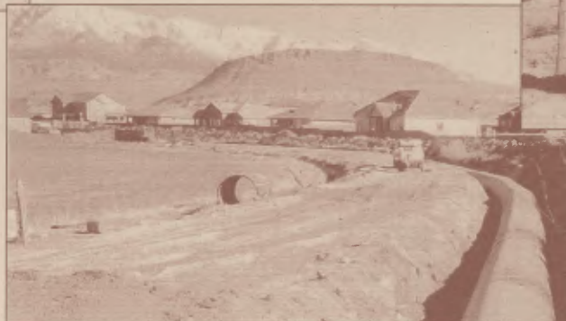
The irrigation canal was put into a pipe in the fall of 2006.
