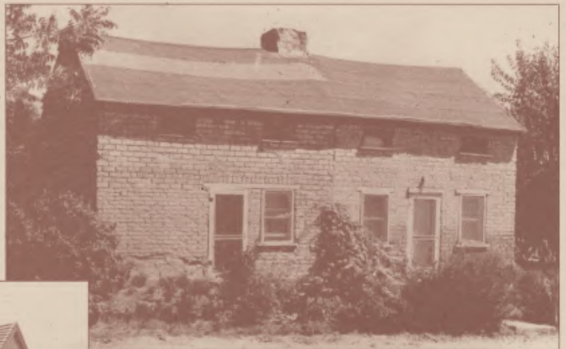
Most of the earlier homes were constructed of adobe since lumber was not easily obtained.
