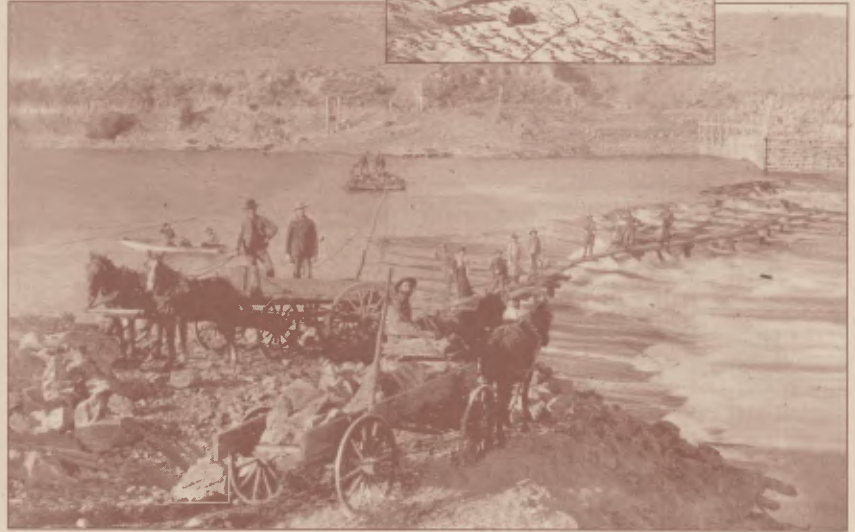
Spillway under construction - completed in 1891
