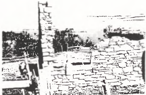
Fig. 7. Ruins of the Wilford Woodruff room in 1956. Top of chimney on left is shown in right background of Fig. 6.
