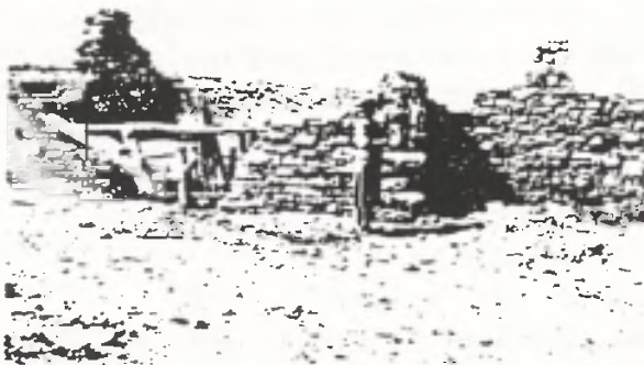
Fig. 6. Ruins of the old home in 1956. Kitchen on left, living room on right.
