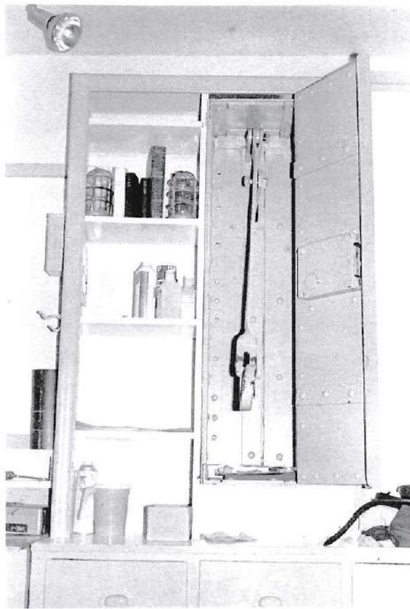
This photograph (dated 01/22/1977) shows this same locking system with the lock open showing the large lever which, when pulled down slid the locking bars across the top of the individual cell doors. The "Tank" cell required a separate key. This allowed the individual cells to be opened but maintained the security of the prisoners.
