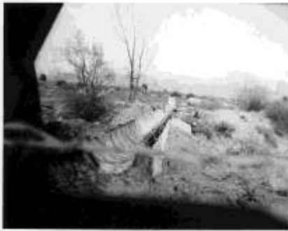
1940's Metal flume built to carry irrigation water over wash to east side of town.
