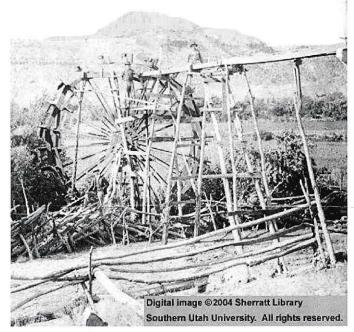
Settlers used other methods to irrigate their land besides the historic canals and ditches. This 1898 photograph shows three men working on a water wheel which raised water from a short feeder canal alongside the Virgin River up to a wooden flume about twenty feet higher than the river which provided water for crops.
