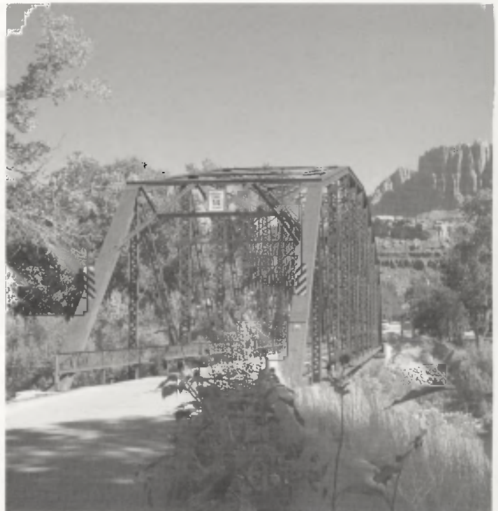
The Rockville bridge looking north.
