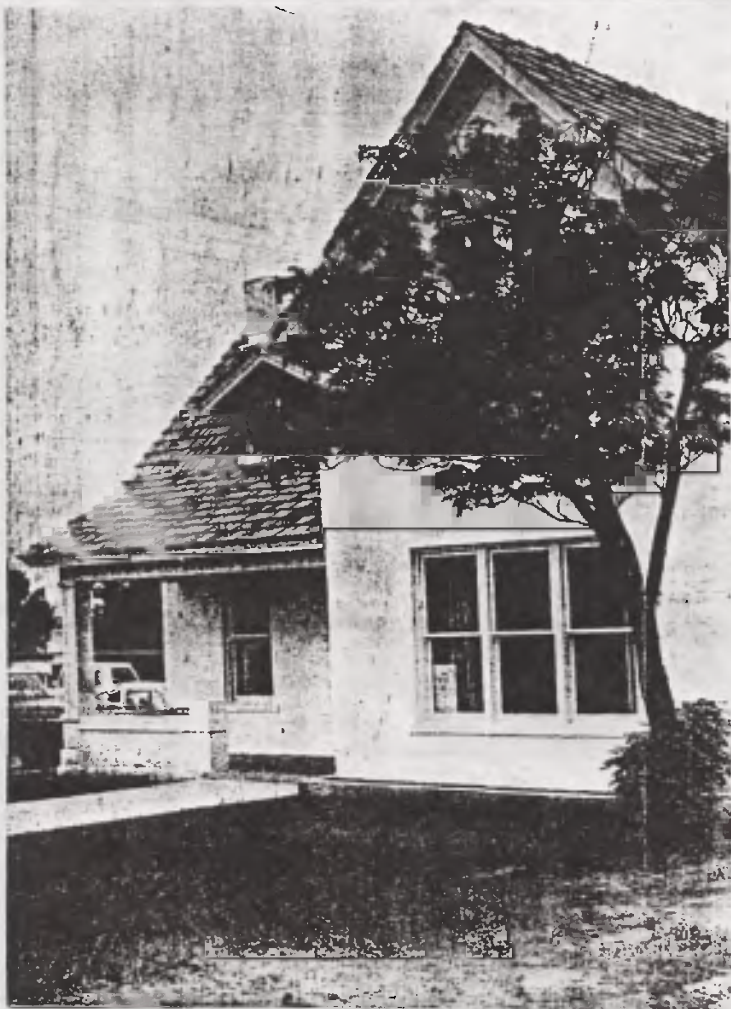
The old A.K. Hafen Home has been remodeled and is now for lease for commercial purposes. Dr. Larry Staples has spent the past eight months in working with contractors in the restoration of the century-old house.
