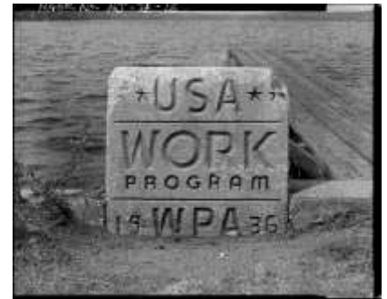
WPA marker, Upper Doughty Dam, Atlantic County, NJ (HAER NJ-78-15)
