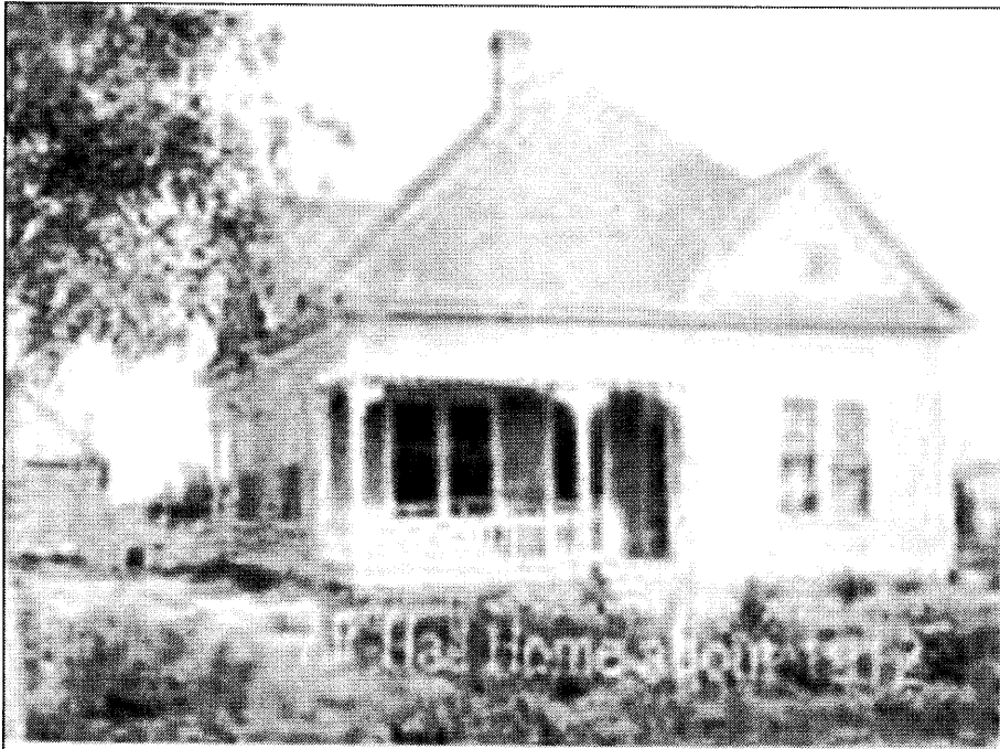
Alfred & Julia Hall Home 1912 was at 200 South 200 West Hurricane, UT
