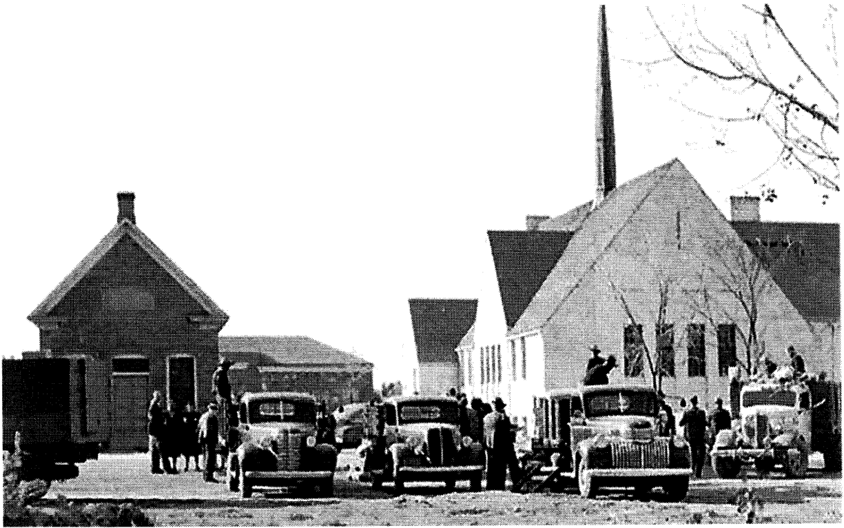
Relief Society Hall - Hurricane High School - White Church - 20 South Main - abt 1937 RS building torn down - HHS demolished 2003-04 - White Church demolished August 1985
