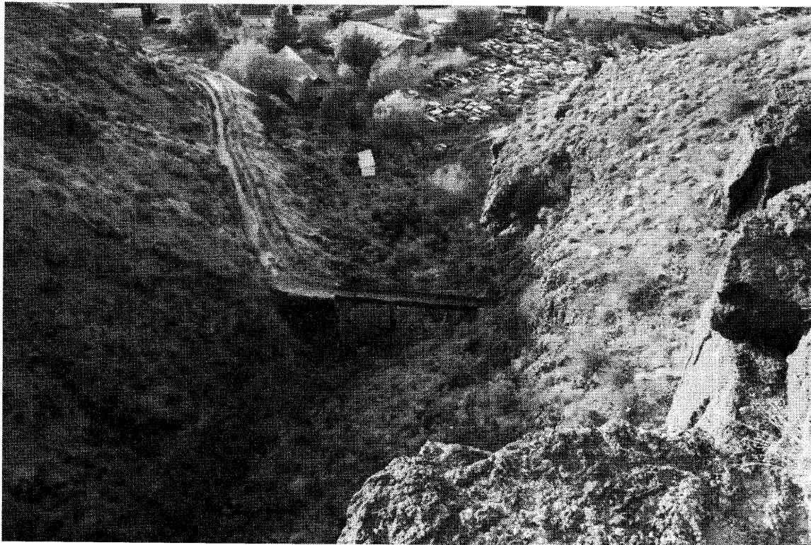
One of the Canal Flumes coming out from a Tunnel
