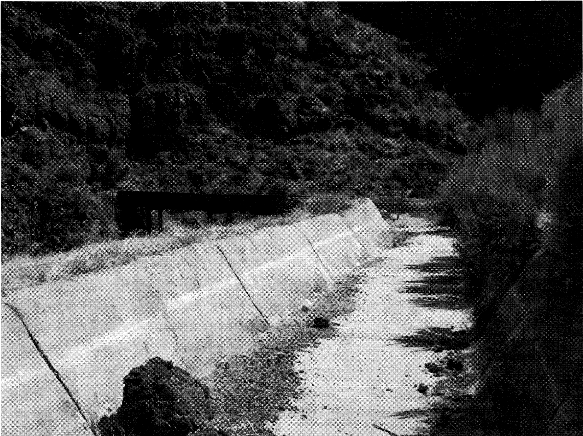
Hurricane Canal (a concrete section)
