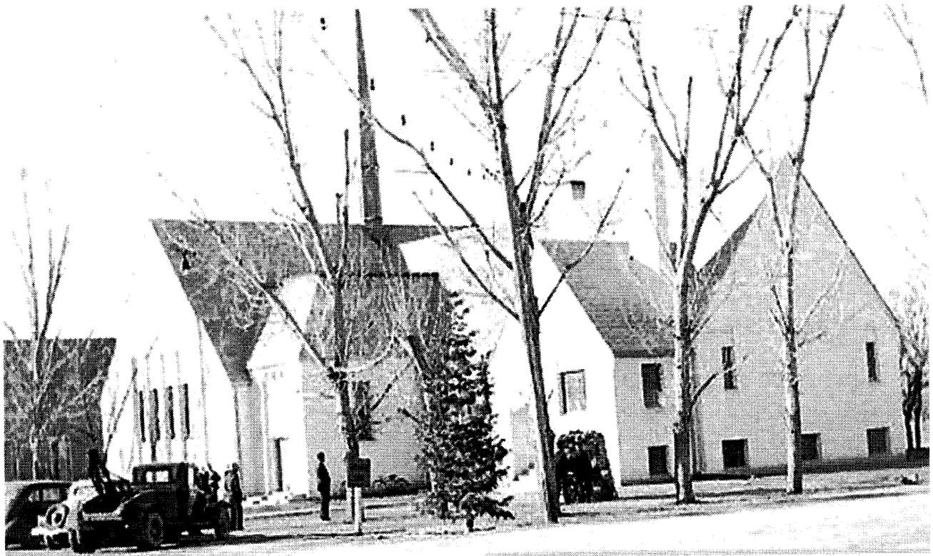
White Church 20 South Main - Hurricane Demolished August 1985
