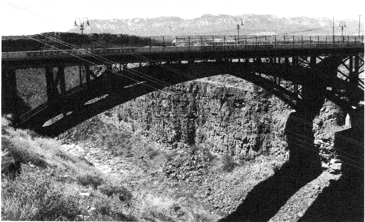
Virgin River Bridge - 1937 - Rehabilitated in 2003 from 2 lanes to 4 lanes of traffic
