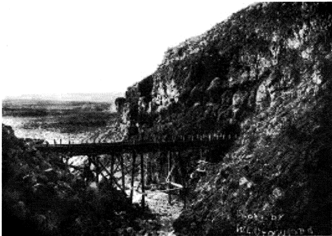
One of the Canal Flumes on a Trestle
