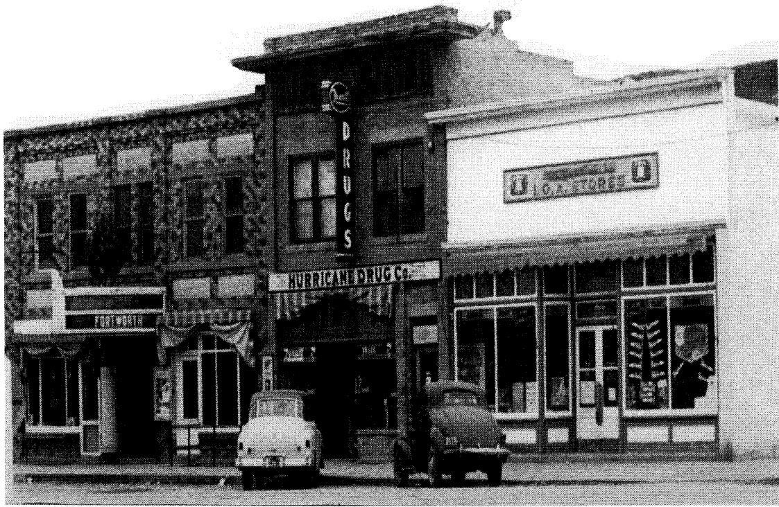
DOWNTOWN HURRICANE -- North Main & State State LtoR: Upstairs Apartments -- Movie Theater -- Drug Store & Ice Cream Shop -- Grocery & House Goods
