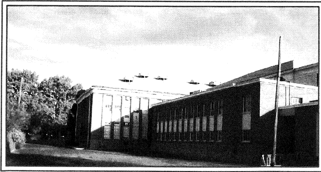
North Classrooms Gym From State Street
